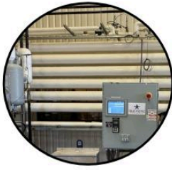
Ice / Cold Air Colocation
