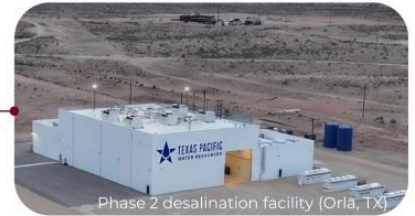
Phase 2 desalination facility (Orla, TX)
